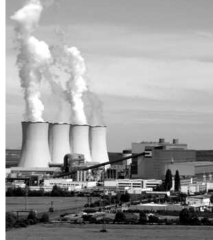
Fig. 2 Tušimice power plant
