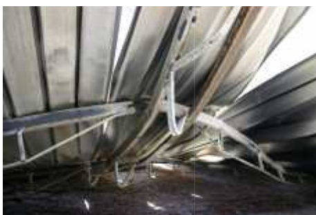
Fig. 9 – Secondary beams instability top chord
