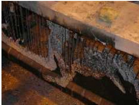
Fig. 4 Beam No. 1 (ref. Mix 1) after failure due to web destruction
