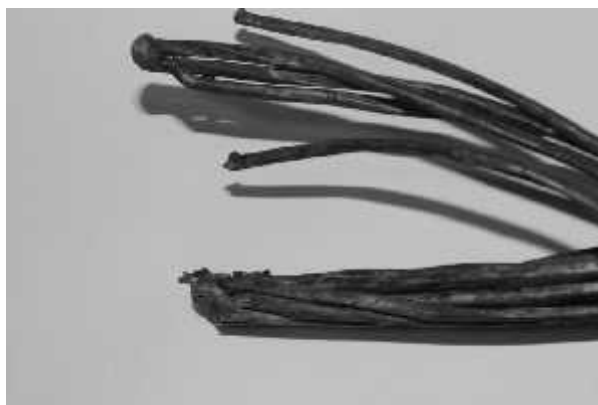
Fig. 6 Traces of the primary short circuit at the end of the conductor
