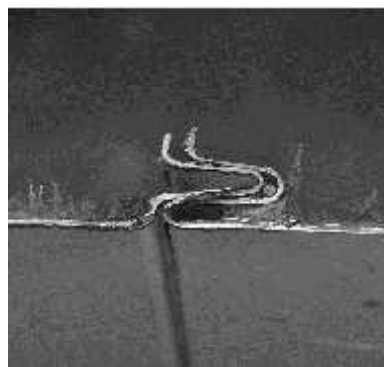
b) Cladding from unexposed side of panel with MW core after the test
