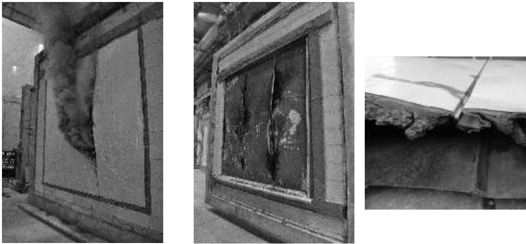
a) View of test specimen during the fire test b) View of test specimen after the test - unexposed side c) View of cross section of panels with PIR core
