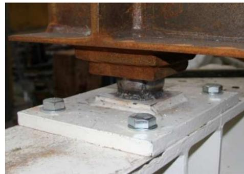
Fig. 4 Fixed pin point support
