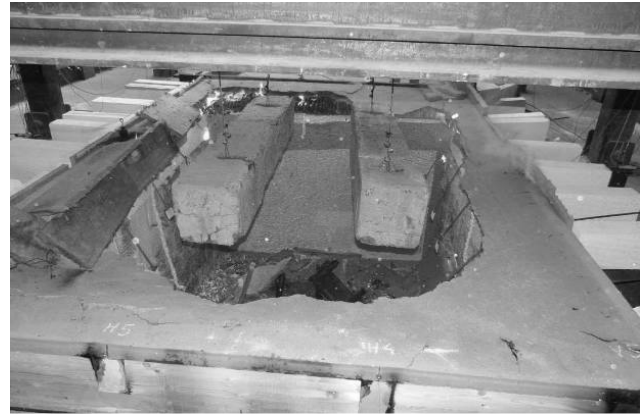
Fig. 3 Collapse of the composite slab
