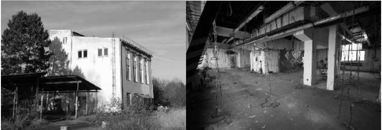
Fig.1 Left – Southwest corner of test building, and Right – fire compartment
