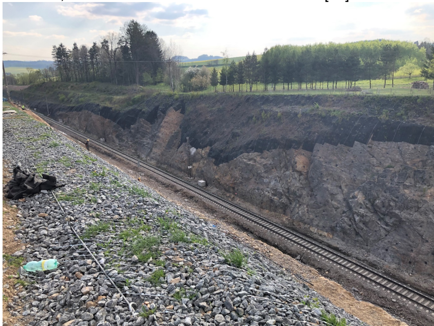
Fig. 4 - Excavation works on the rock cut slope (Author)
