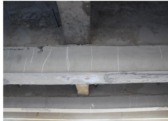
(b) - Composite mortar crack diagram
