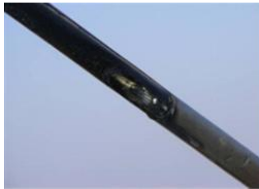
Fig.1 - Fire diagram of two back cables on the downstream side of the north bank
