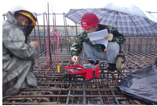
Fig.14- Strain test diagram of main girder
