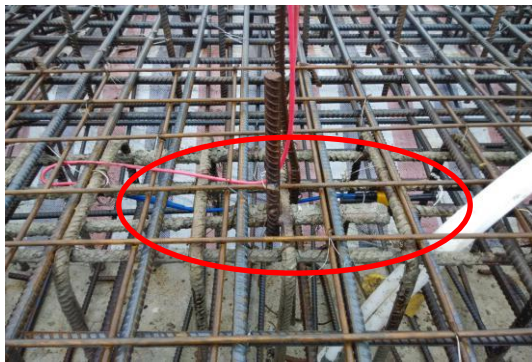
Fig.13 - Main girder strain gauge installation diagram
