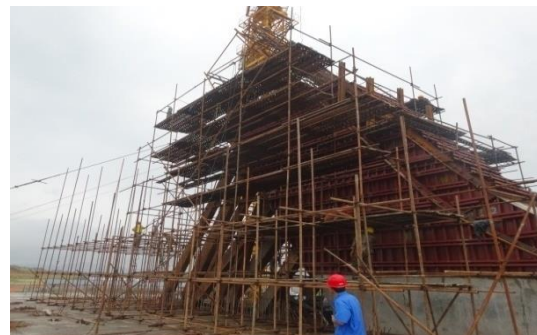
Fig. 4- Tower turning mold construction
