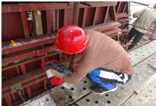
Fig.15-Strain test diagram of bridge tower
