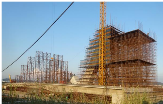
Fig. 3 - Cable tower and arch rib support
