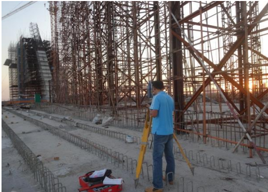
Fig.18 -Main girder elevation measurement anchor point
