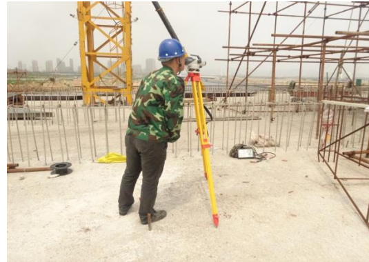
Fig.19 -Tower elevation measurement diagram
