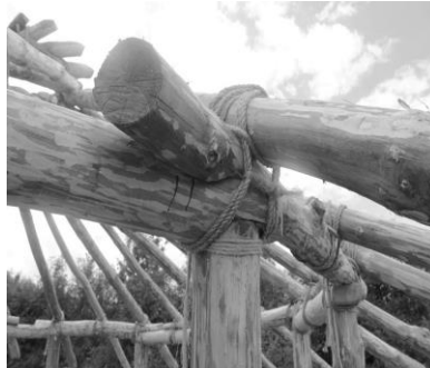
Fig. 4 - Lashed connections
