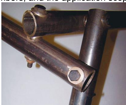
Fig. 6 - Bolted connectors
