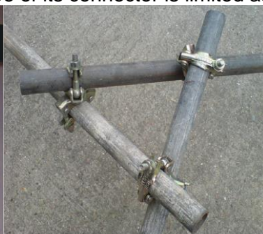
Fig. 7 - Scaffolding swivel couplers
