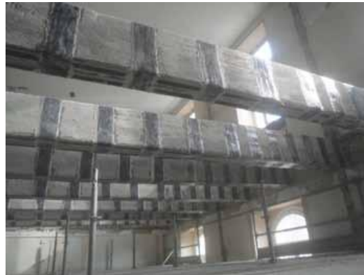
Fig. 1 – FRP sheets bonded to the external surface of RC beams
