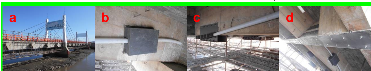
(e) Photo of the strengthened structure
