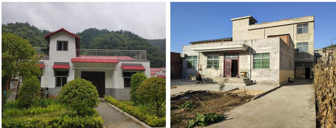
(a) A self-built house designed and built by Shangluo municipal government
