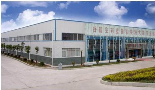
(c) Steel frame workshop
