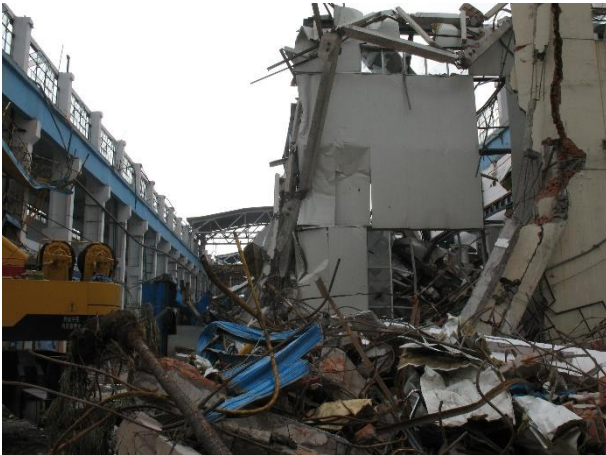
(e) Overall failure of MS and steel frame industrial building
