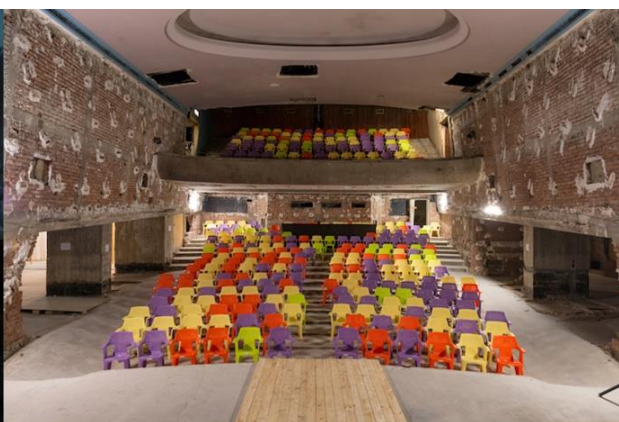
Fig. 7 - Auditorium of the cultural space 64 U Hradeb during reconstruction [25]
