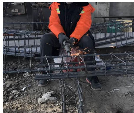
(b) Rebar grinding
