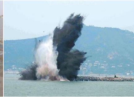
*Fig.3 - Blasting compaction*
