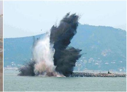
*Fig.3 - Blasting compaction*
