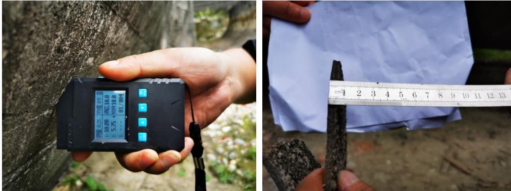
Fig. 3 — Detection of carbonization depth of Jigongzui aqueduct body
