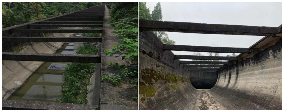
Fig.1 — Current situation of Jigongzui U-shaped thin shell aqueduct project
