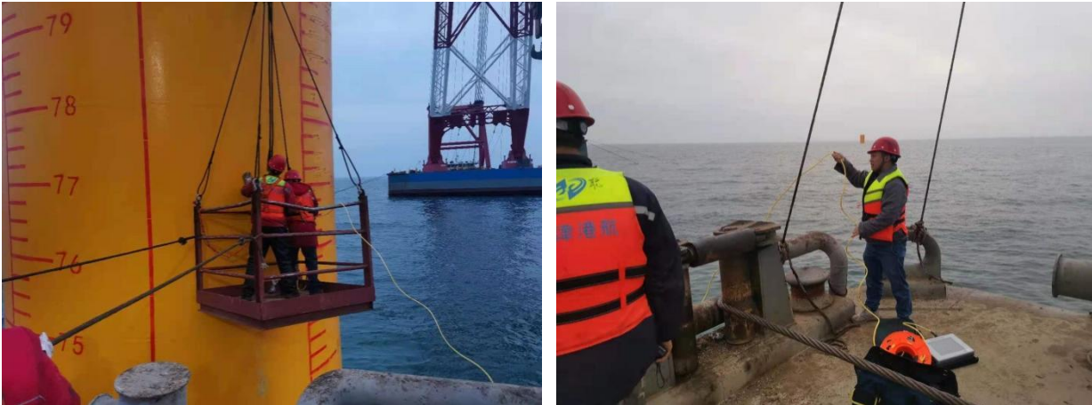
Fig. 1 – High strain detection of large-diameter monopile
