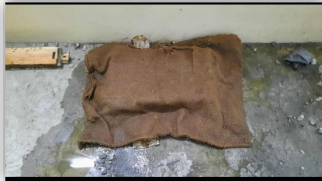
Fig. 4 – Curing of Slab using Jute bags
