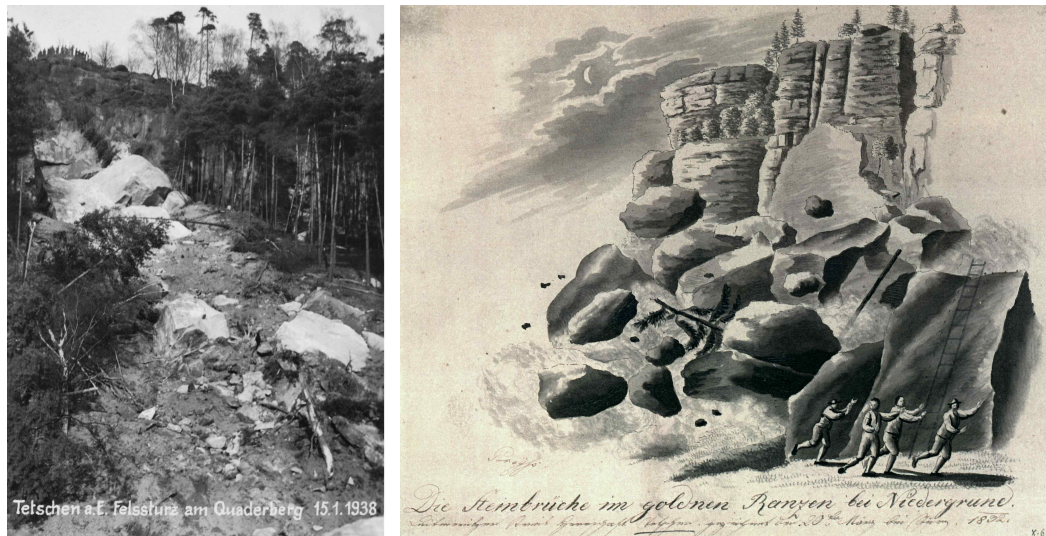
Fig. 3 - Left: A historical photograph of rockfall in a quarry at Kvádrberk Hill in 1938 (archive of P. Joza); Right: A wash drawing by J. Preyss, the parish priest of Hřensko, showing the rockfall of March 20, 1832 in the Goldenen Ranzen Quarry (near the Suchá Kamenice River); then, blocks at the foot of the slope were quarried by wedging, and a spontaneous fall of the quarry face occurred in the upper part of the slope (collections of the Municipal Museum of Ústí nad Labem)
