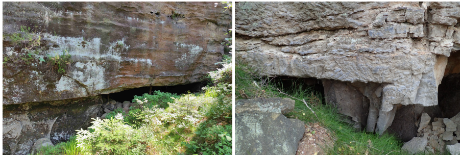
Fig. 2 - Unfinished mining using the undercutting technique in the Elbe River canyon: left) in the area of the Comiteebruch Quarry, preserved as a deep “overhang” 7×3 m in size; right: unstable rock wall in the whetstone quarry near Podskalí (photo by Z. Vařilová)
