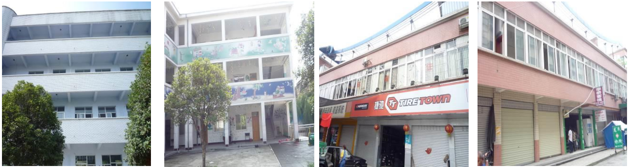
Fig. 11 – RC frame structure after seismic design basically intact
