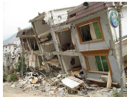
(b) Ensemble collapse of bottom layer
