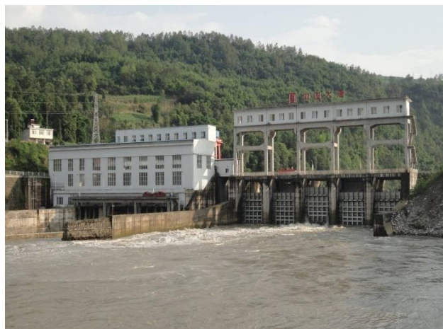
Fig. 2 – Site photos of Xinzhong Hydropower Station
