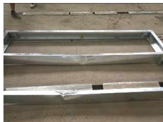
(g) – Destruction of steel frame
