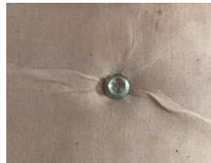
(b) – Sinking of self-tapping screw
