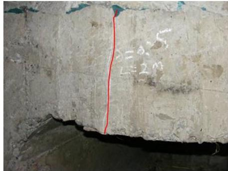
Fig. 4 – Crack on interior diaphragm of box girder end of the first span
