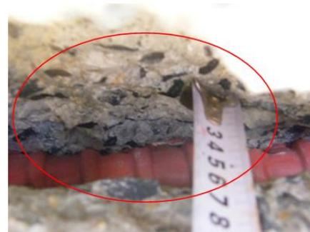
(f) longitudinal crack corrugate pipe deterioration of second span
