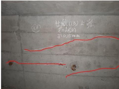
(e) No. 13 block right side interior surface crack (L=6.7m δ=0.15mm α=45°)
