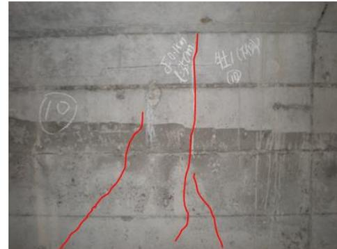
(f) No. 10 block left side interior surface crack (L=2.9m δ=0.10mm α=45°)
