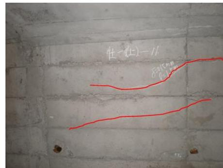
(d) No. 11 block left side interior surface crack (L=3.4m  $\delta$ =0.15mm  $\alpha$ =30°)
