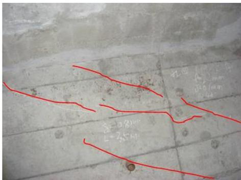
(c) No. 10 block right side interior surface oblique crack (L=9m  $\delta$ =0.5mm  $\alpha$ =35°)
