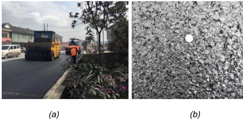
Fig.11 - HMA pavement after construction
