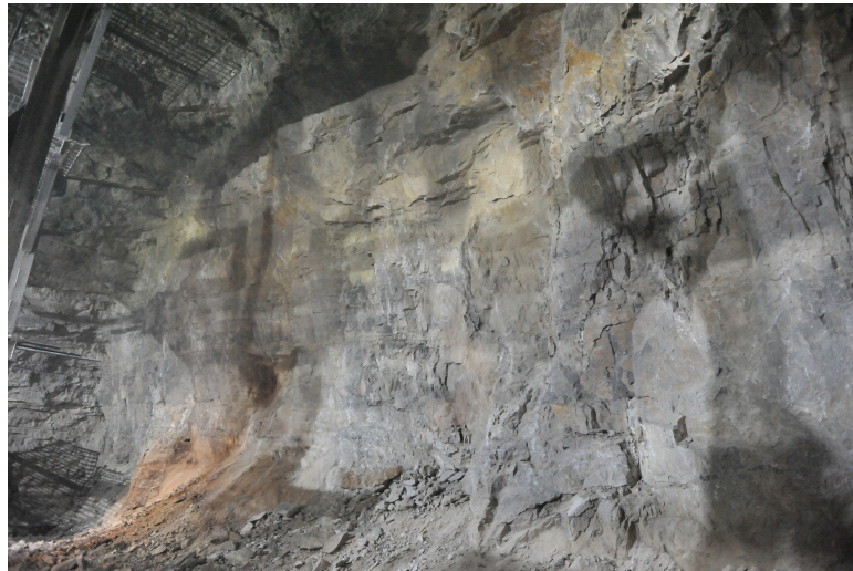
Fig. 4 – Monitoring section rock condition
