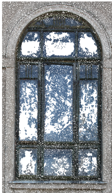
Fig. 7 – Example of the second window type - section from point cloud
