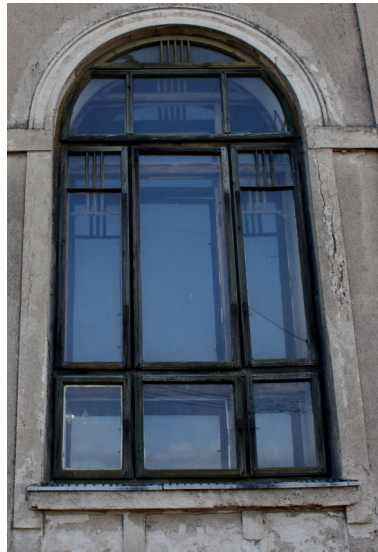
Fig. 4 – Example of the second window type - section from the photo
