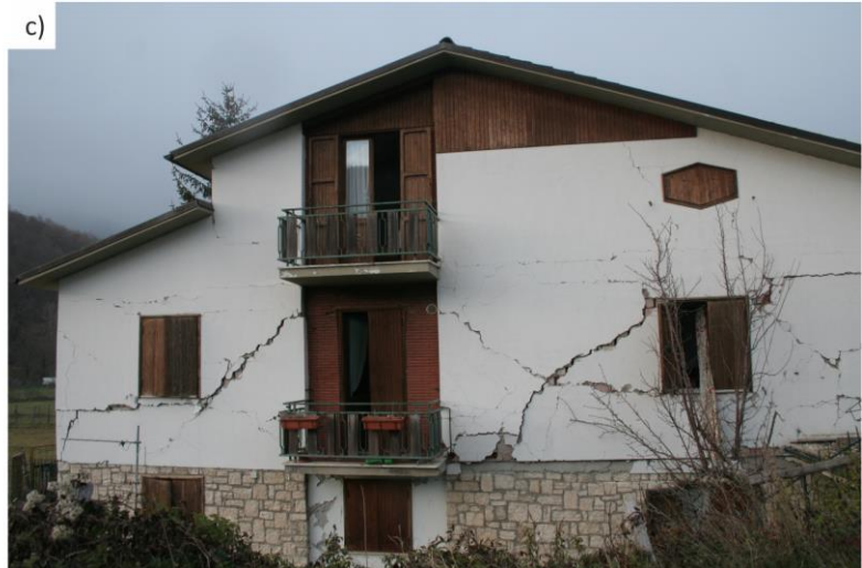
Fig. 8 – Failure scheme of masonry buildings due to dynamic effects, a) Pile driving, b) Blasting, c) Natural seismicity
