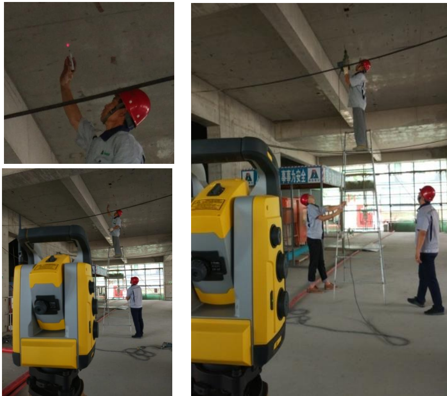
Fig.8 – Positioning robot application
