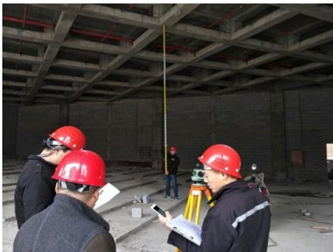
Fig. 8 – Pictures of on-site measurement of the first-floor slab
