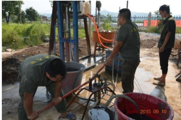
Fig. 9 – Picture of grouting process
