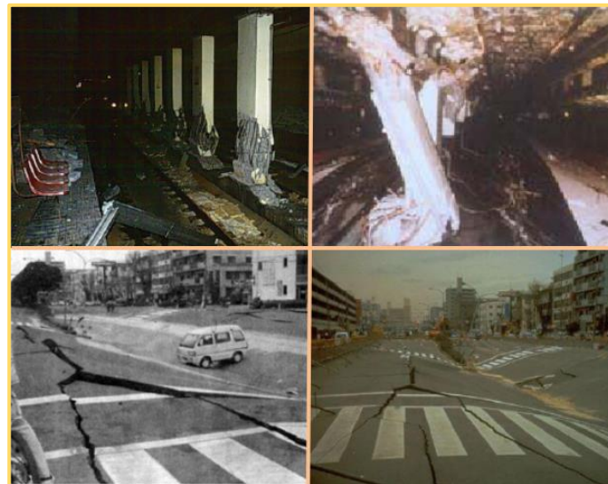
(a) Earthquake Damage of Dakai metro station [13]
