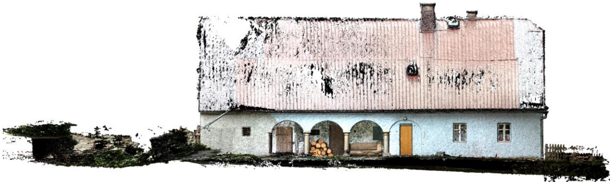
Fig. 10: Example of the point cloud, front view, Stříbrnice (Šumperk District, Czech Republic)
