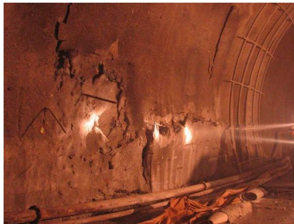
*Fig. 1 - Liner failure caused by rock slide along fault [7]*
