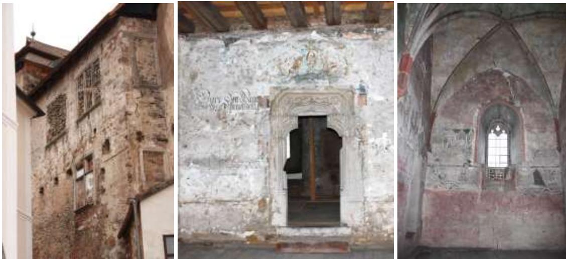
Fig. 1: Bečov Castle – authenticity of plaster surfaces: a) southern facade, b) the Annunciation Chapel, c) corner room in the donjon) stress the genuine historical appearance of buildings
