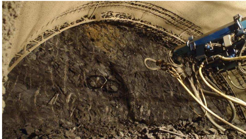
Fig. 2. Face anchors installation, Veleslavín Station, Czech Republic (author's archive)
