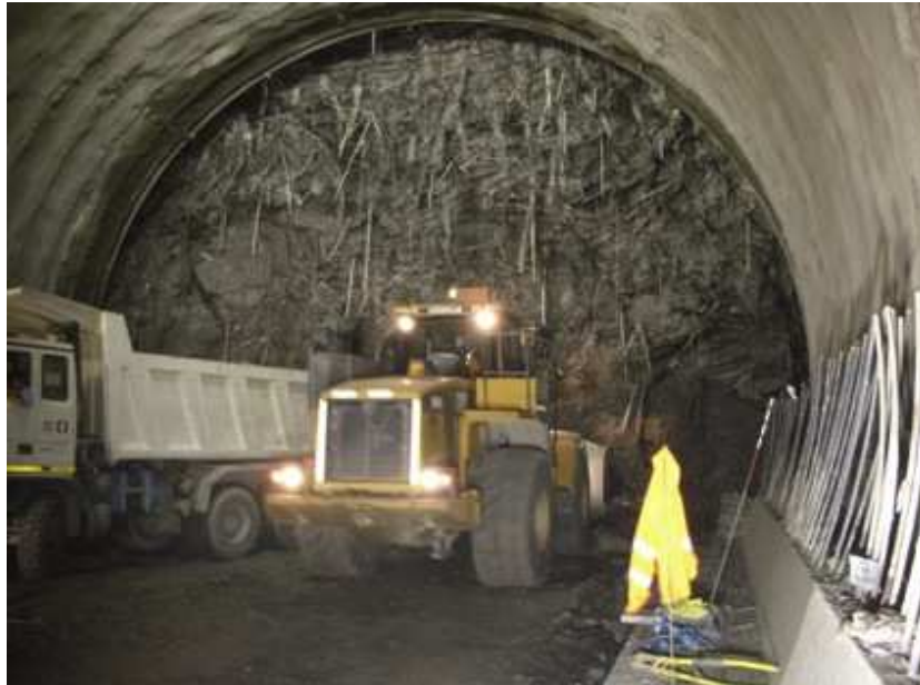
Fig. 3. Excavation process, Val di Sambro Tunnel, Italy (author's archive)
