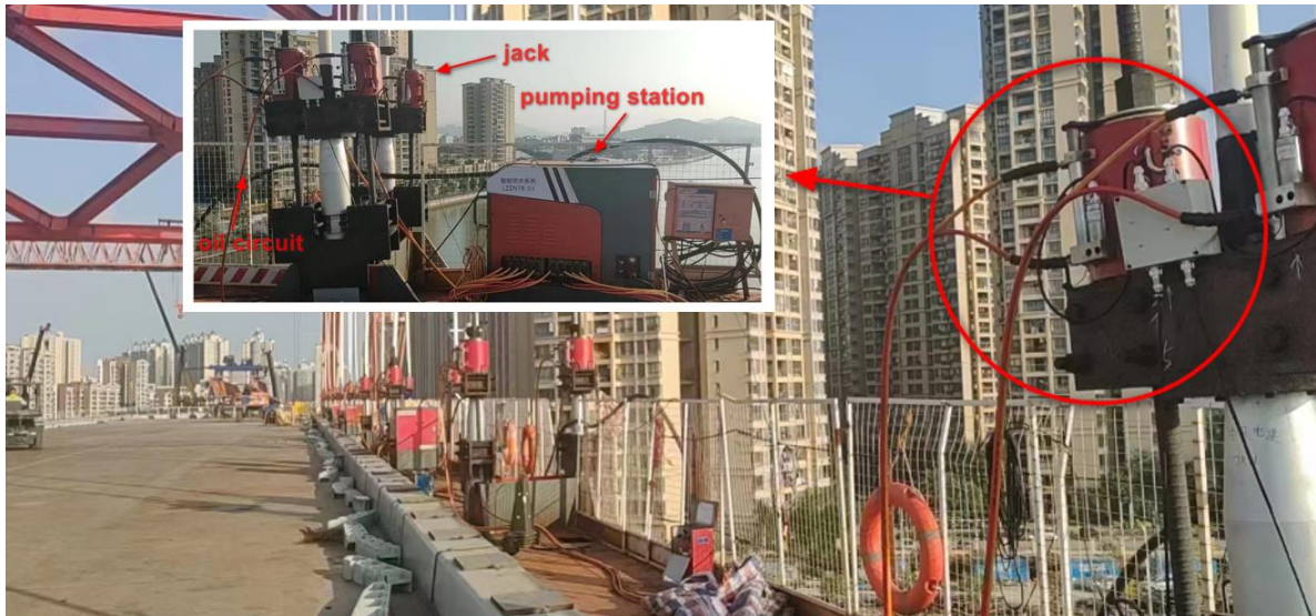
Fig. 5 – Application of integral intelligent synchronous tensioning technology in this bridge
