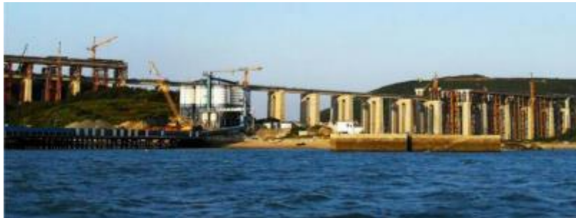
Fig. 1 - Construction site of highway-railway bridge at Pingtan Strait of FuPing Railway
