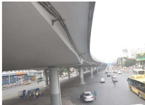
Fig. 1 – Aerial view of the elevated bridge
