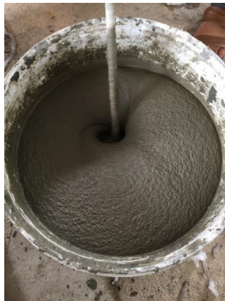
(a) Prepare foam concrete
