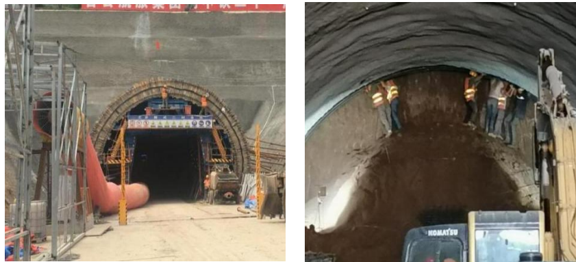
Fig.1- Tunnel scene pictures
