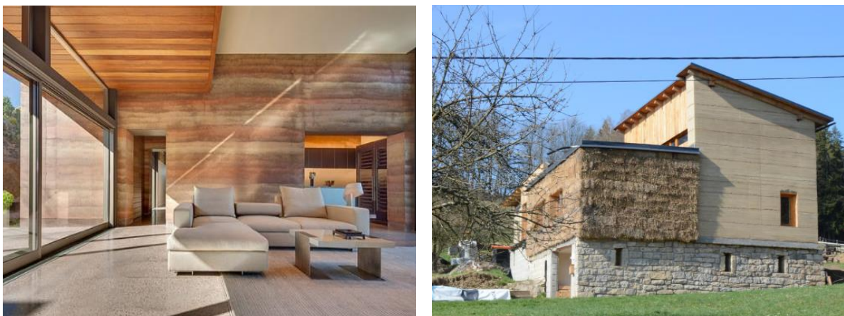
Fig. 1 – Modern rammed earth buildings: on the left, a house in Santa Fe [11] and on the right, in Plavy [12]
