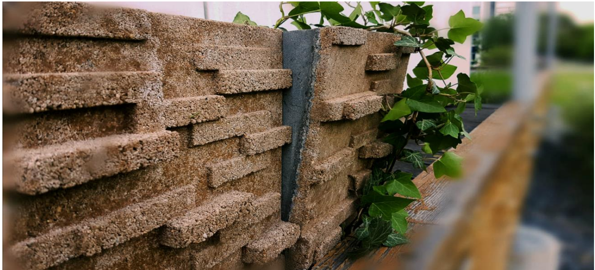
Fig. 12 - Prototype tile produced using the optimized mixture - outdoor installation
