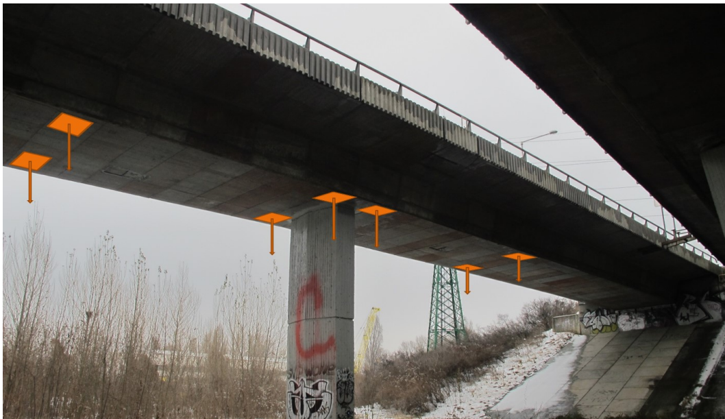
Figure 3: Vertical displacement determination of part of the Harbor Bridge in Bratislava
